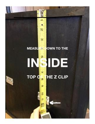
3. Mark the top of the Z Clip opening location on the wall, place first Z Clip in the location you want, and mark the two holes. Repeat process for second clip.
